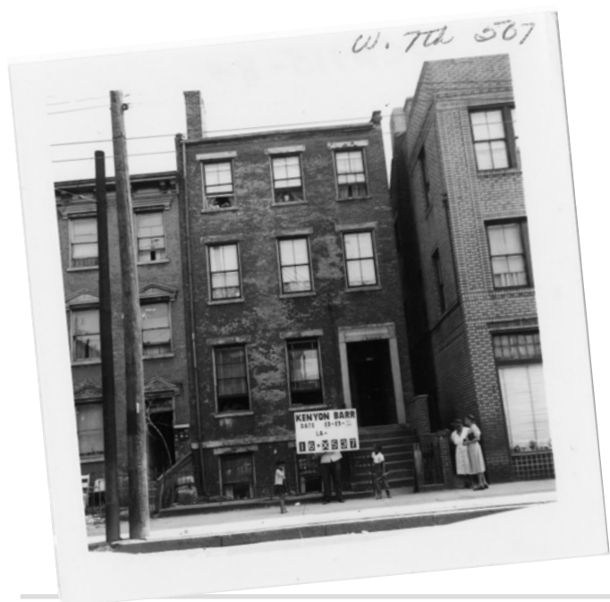
507 W. 7th Street. 05/05/1959. Structure at 507 West Seventh Street.
