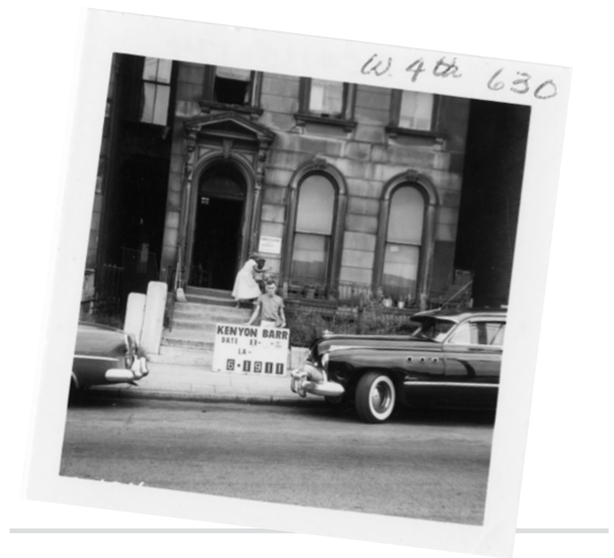
630 W. 4th Street. 08/01/1959. Structure at 630 West Fourth Street.
